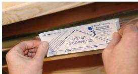
**2. Cut out the triangle.** Drill a 3/4-inch hole at each of the 3 corners and connect the holes with your snips.
