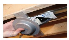
**4. Twist into position.** After the blade is inserted, rotate the damper 90° with the tubing port facing the main duct.
