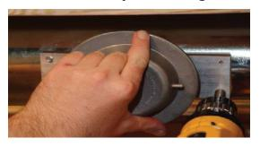
**6. Attach the air line.** Cut a 3/4-inch section out of the "homerun tube" for that zone and insert a tee to connect to the damper.
