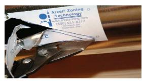
**3. Insert the damper.** Hold it in the closed position, and insert the blade at the wide end of the triangle.
