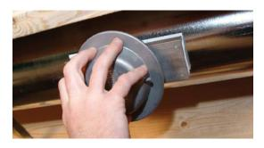
**5. Fasten with zip screws.** Secure the damper at two opposing corners. Add the other two screws. Tighten all four screws to just seal the gasket.
