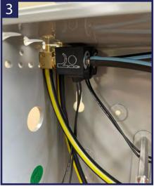
Insert the provided solenoid, and mount it into a space at the corner of the panel using two of the provided screws. Ensure that port #2 is pointing out of the panel. Connect the tubes from step two as shown.
